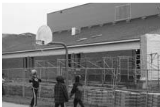
Exterior progress on the JH wing
