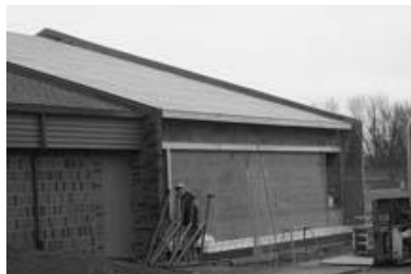
Exterior walls of the elementary addition
