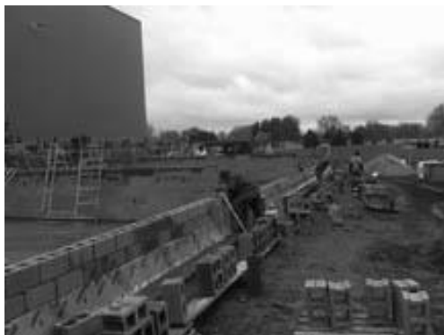
Beginnings of the work being done
